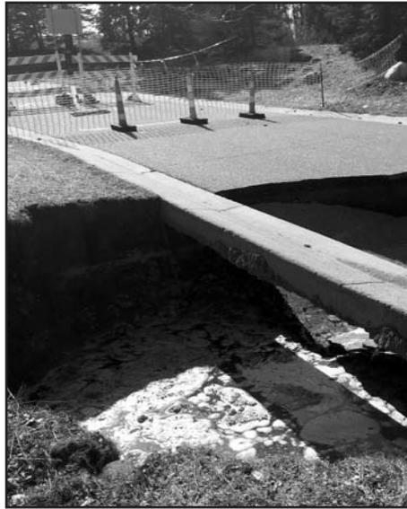
*The sinkhole was created when water from the failed culvert washed out soil under the road. This left the pavement unsupported, and it collapsed.*
