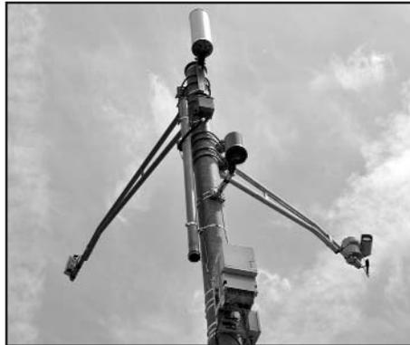
*The small cell hardware on an RCOC pole.*
